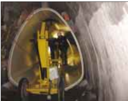
HOBAS NC Line pipe installation
