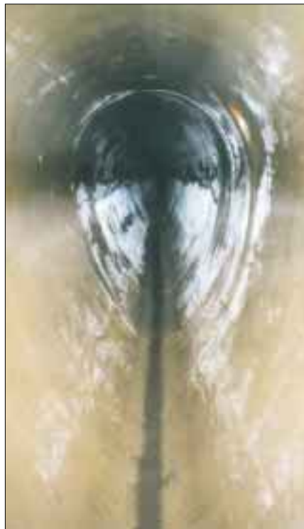
Rehabilitated sewer with DN 200 laminated inlet
