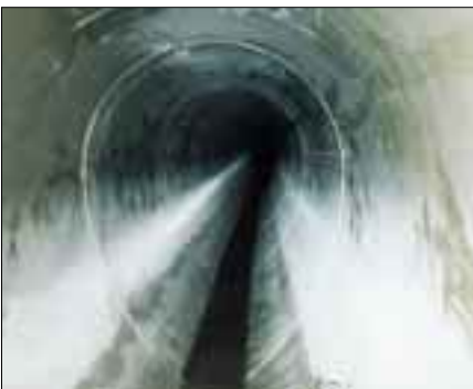
View into the rehabilitated sewer.
