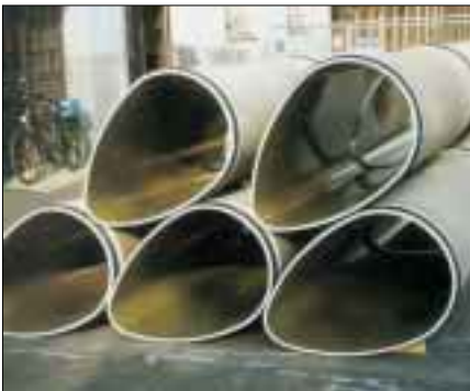
The DN 680/1050 relining pipes stored in front of the access shaft.
