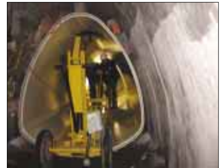
HOBAS NC Line pipe installation
